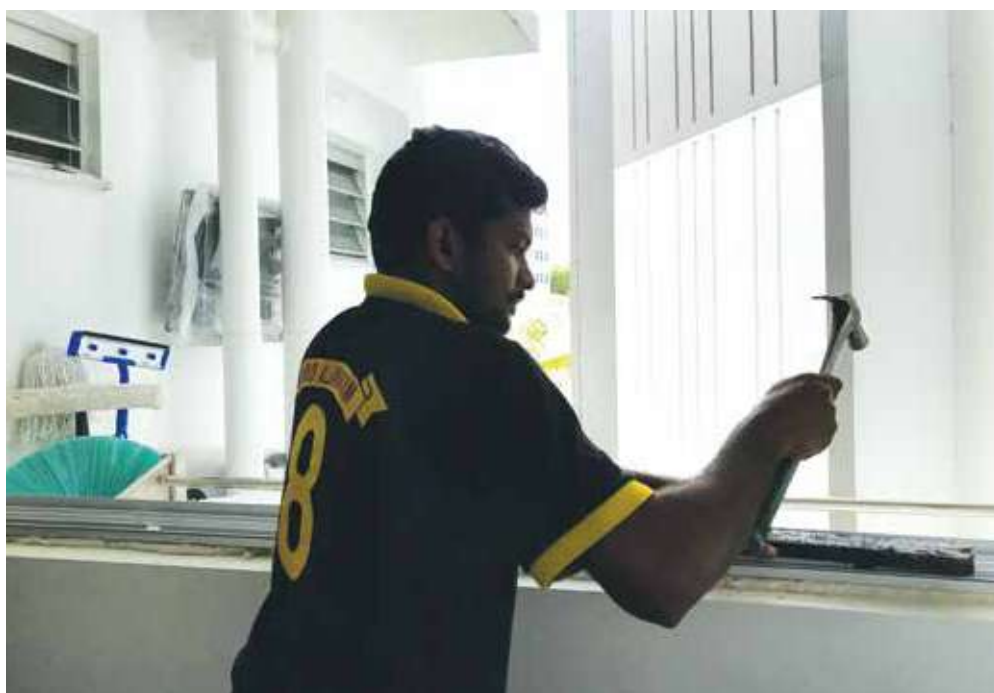
Installing sliding windows at the service yard
